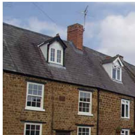
Rectangular brick chimney at edge of mid-terrace dwelling, central to gable, Adderbury
