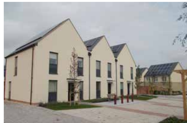
A shared surface street - NW Bicester
