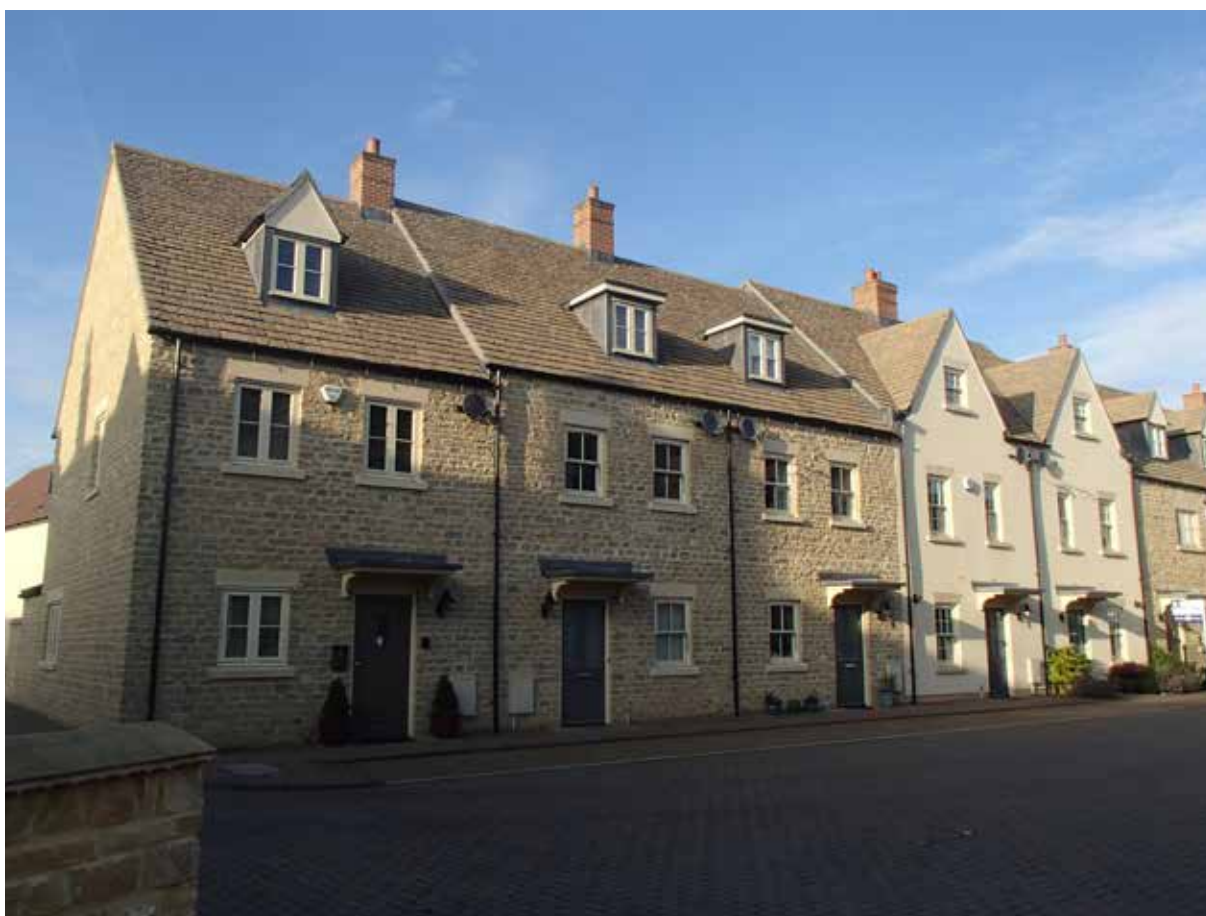
The use of locally appropriate, high quality materials must be considered early on - Ashford Close, Woodstock
