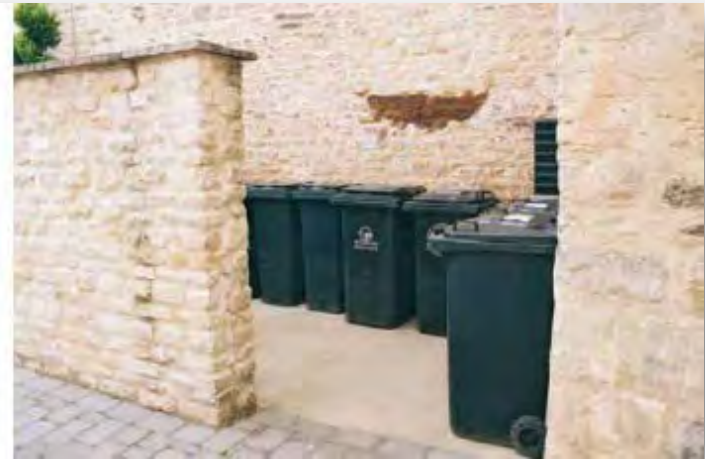
Attractive bin store with appropriate materials. Images from West Oxfordshire Design Guide
