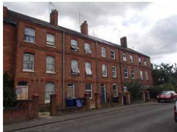
Narrow fronted 3 storey terrace, Banbury
