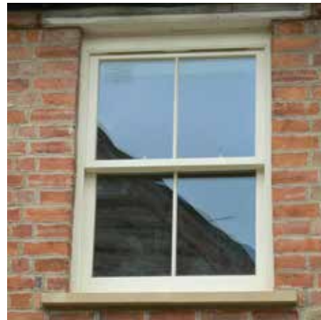
Sash window, Woodstock
