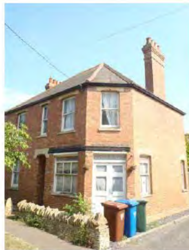
Cutting off edge to address corner, Islip
