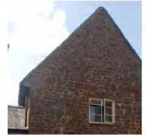
Roofs and eaves
